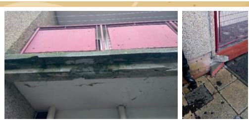
This will involve taking the concrete back to a solid stable state and new reinforcement bars being inserted and a new front to the balcony being formed. We have successfully carried this out at Cheviot Crescent and Longhaugh Road in the last year (see image in article above).
